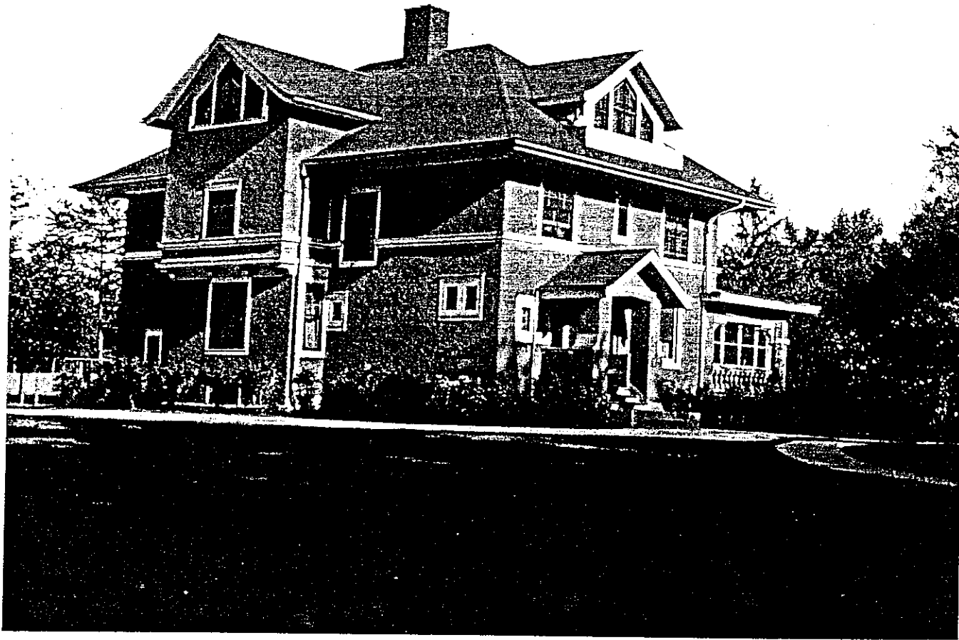
Pentecost House, historic photograph post 1910
