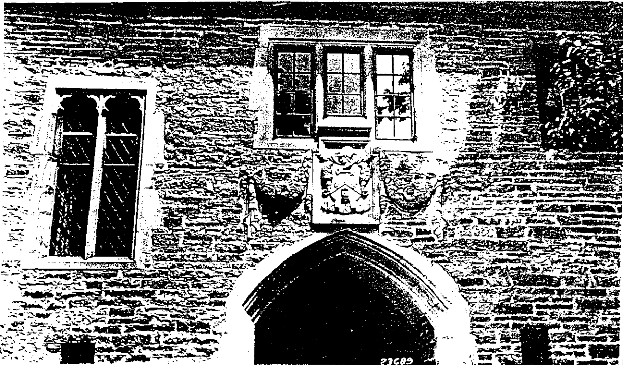
Kappa Kappa Gamma Fraternity House, 1102 S. Lincoln Ave., Champaign, Illinois. Urbana, IL Howard Shaw Associates, Architects. 1928
